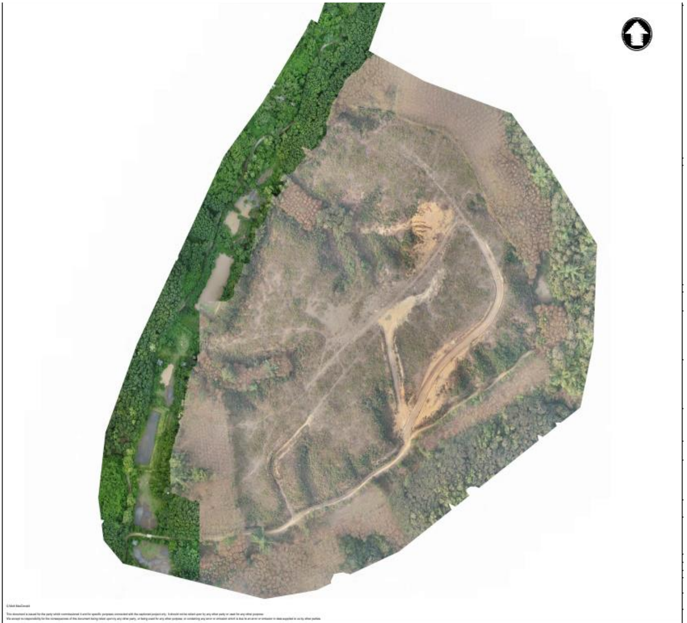
Figure 2: Drone image - aerial view of Nagicherra Industrial Estate
